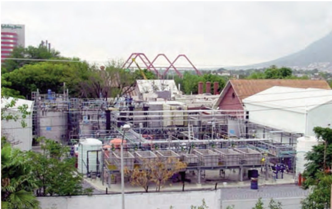
Fig. 8. A view of Peñoles bioleaching plant in Monterrey in Mexico.
